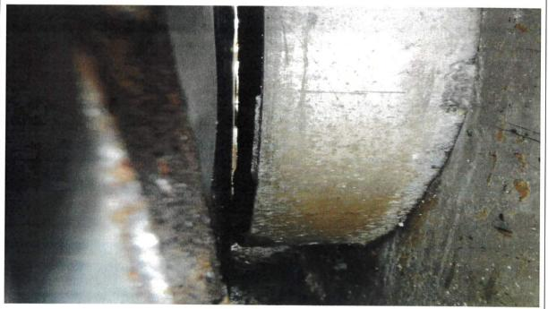
The second picture above shows gate #3 and space between the gate's flapper and the gates frame. The gate flapper would not seal against the frame. The gap was an estimated %" to %".
